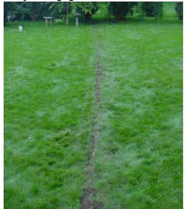
No Mess, No Fuss, Just clean trenches - No Clean Up
