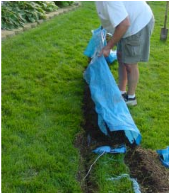
Drop the dirt into the trench
