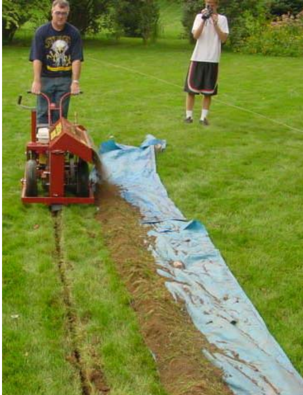
Blows the trenched material directly onto tarps
