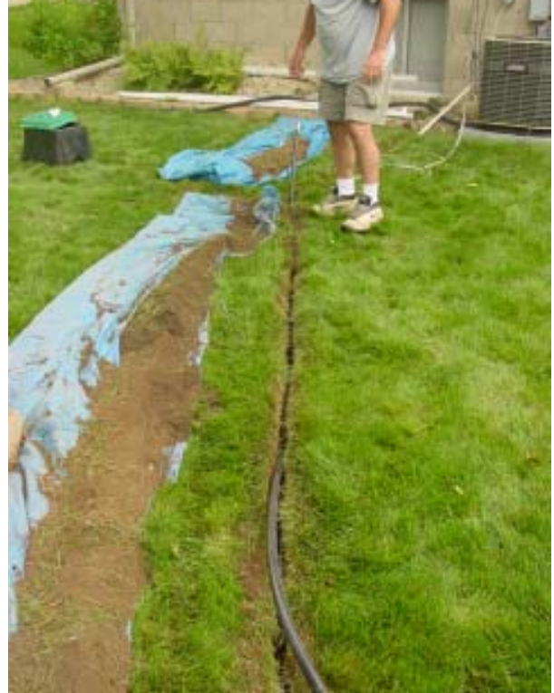
Lay the pipe into the trench
